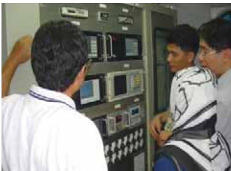
Malaysian public officials inspect the smokestack TMS
